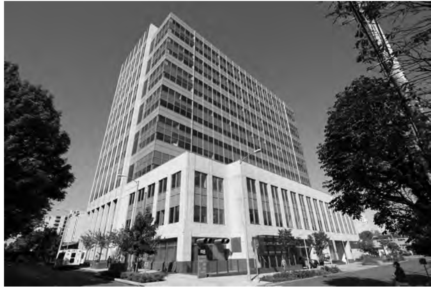
Harborview Medical Center Ninth and Jefferson Building
